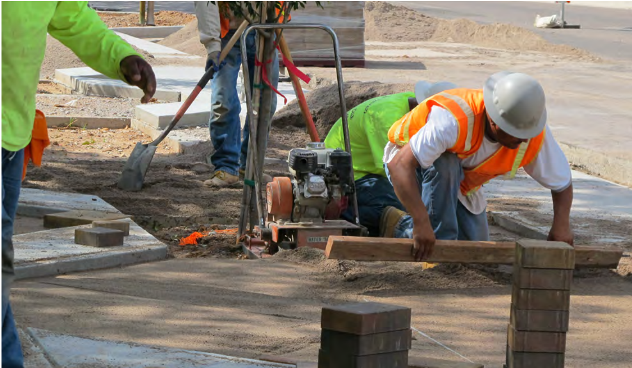
FIGURE 3-12: ACCENT PATH CONSTRUCTION IN DOWNTOWN CHANDLER
