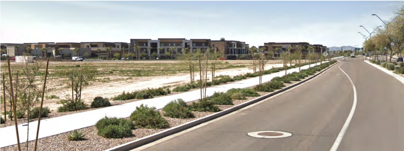
FIGURE 1-40: VIRGINIA AVE EAST OF THE ROOSEVELT CANAL- SOUTH SIDE
