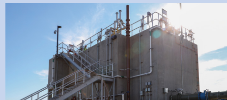
Sand ballast infrastructure at the Surface Water Facility is essential for removing particles during the treatment process.
