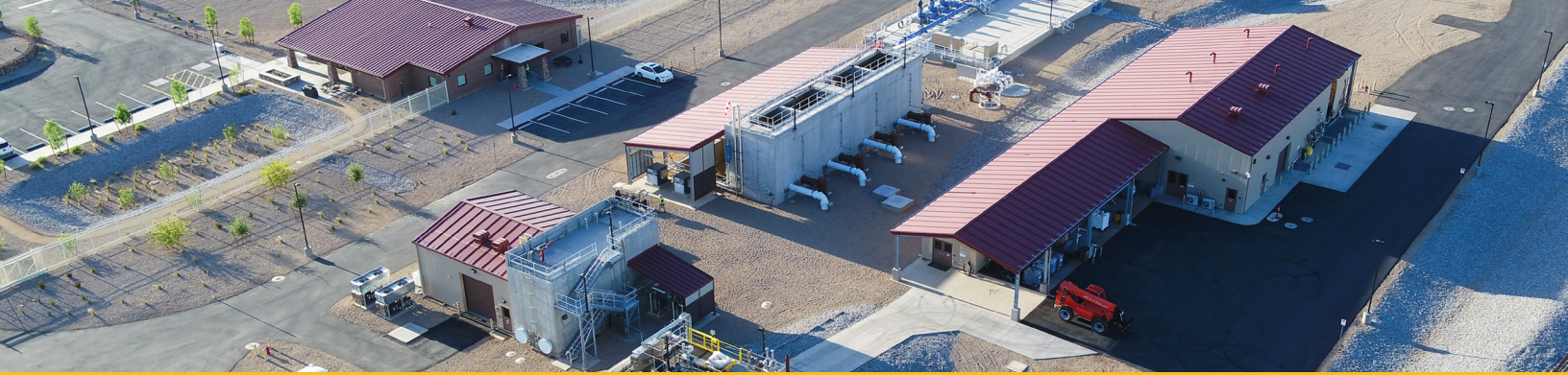
Goodyear's Surface Water Facility where Colorado River and Salt River water is treated for delivery to homes and businesses.
