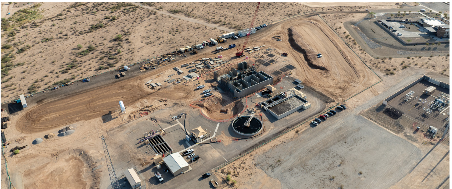
Expanding the Rainbow Valley Water Reclamation Facility in southern Goodyear will help support the city's continued growth.
