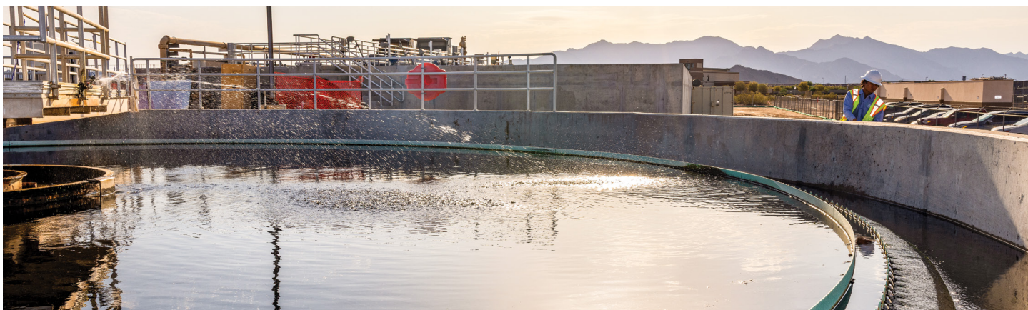
The Rainbow Valley Water Reclamation Facility treats and reuses water, helping expand Goodyear's local water supply.
