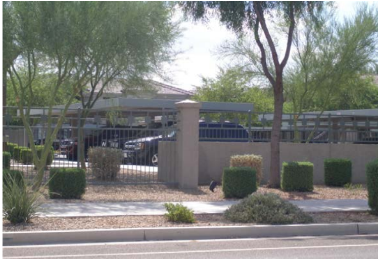
Example of a multi-family development perimeter wall
